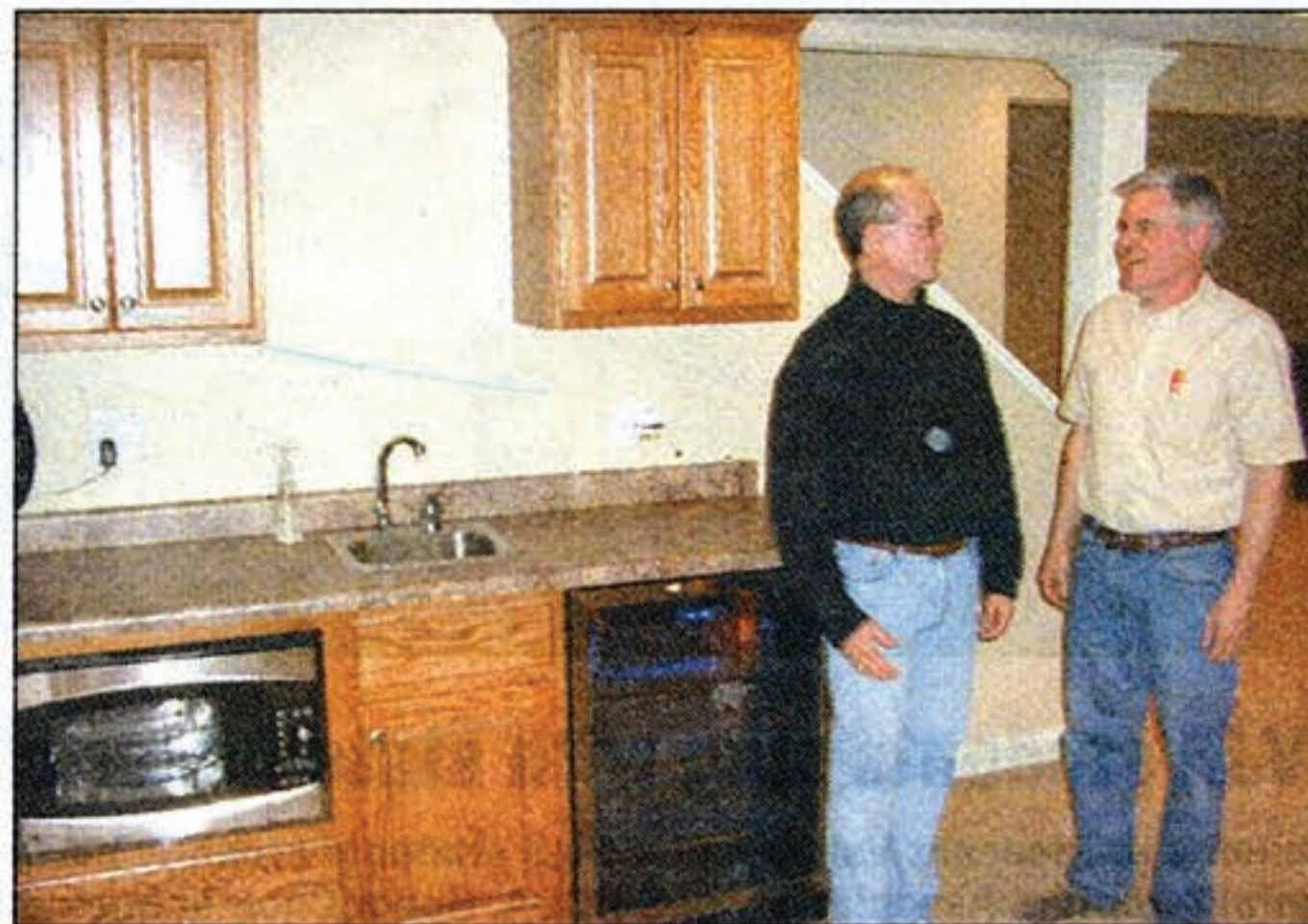
Skip Cramond, left, had contractor Tim Carr put in a kitchenette for quick snacks while watching television or playing games.
